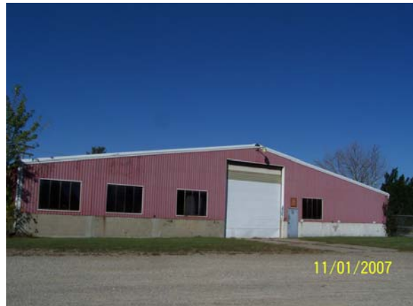
Picture of 9,216 SF truck service building located at 225 Manning Street, Newark, OH.
